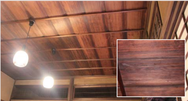
1階「次室」の天井、杉張桁天井
